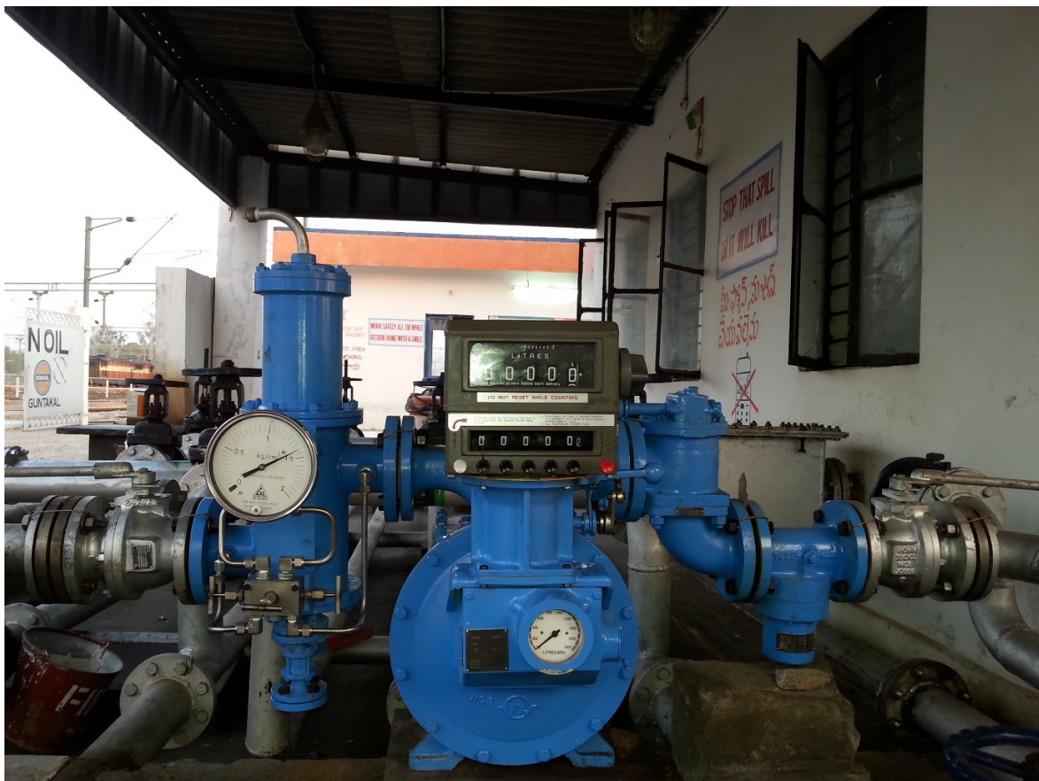
3" P D Flow meter in operation at one of the RCD location.
