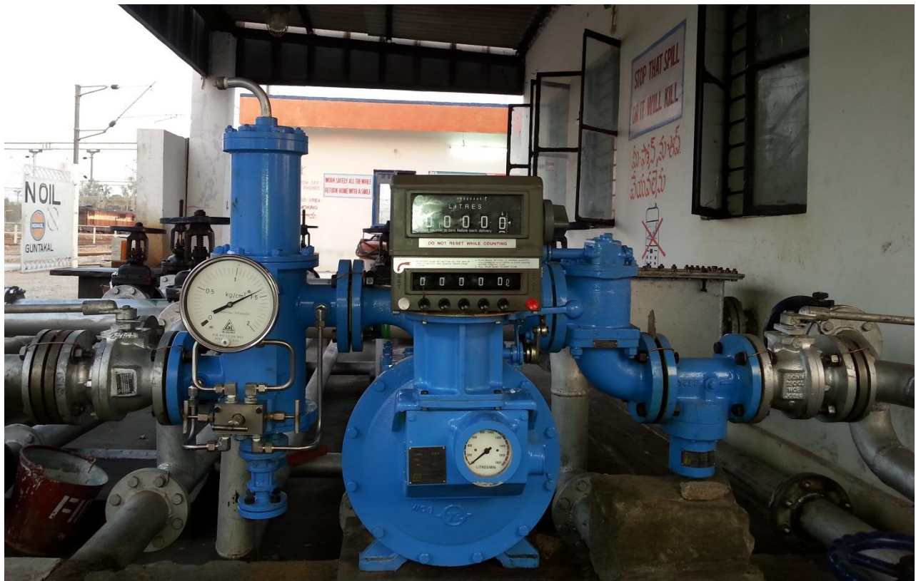
3" P. D. Flowmeter in operation at RCD location
